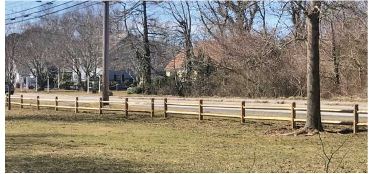
New fencing along Route 6A
