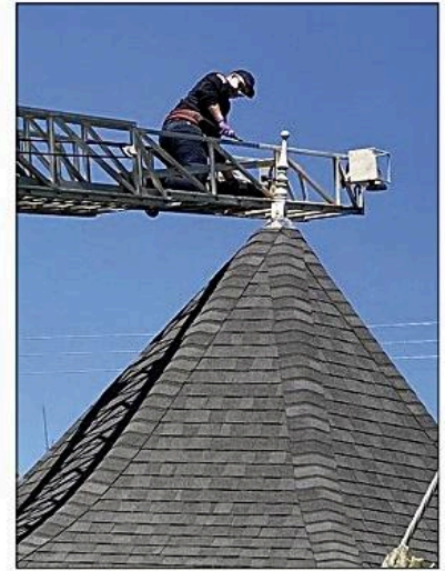
Dennis Fireman from Station 2 putting final touches on the bandstand finial
